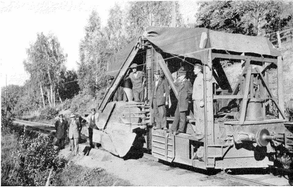
Figure 3—Cable Plough Used in 1924 for the Stockholm-Gothenburg Cable.
